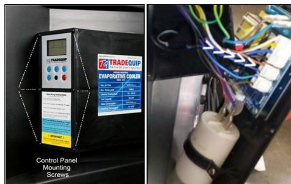
3. Inspect the pump cable plug for loose connection or damage to the plug and socket.
